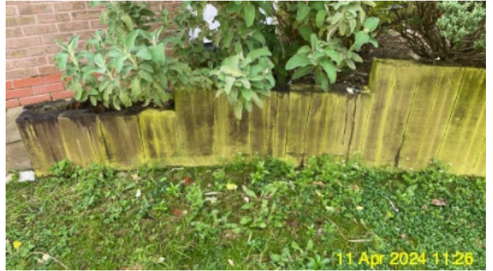
Rear garden/yard (fences, gates, drainage etc)
