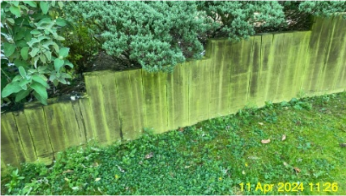
Rear garden/yard (fences, gates, drainage etc)
